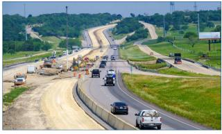
This photo shows road base construction for new lanes and work on widening the Nolan Creek bridge, 7 miles west of I-35.
